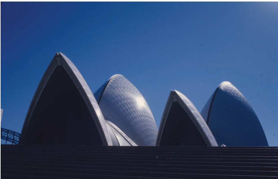
Figure 2 The white tiled roofs of the Sydney Opera House, 1957-1973, reflect the sky. (PD 3057).
