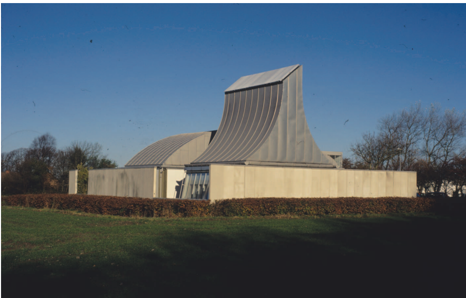
Figure 6 The Utzon-Huset or experimental house, at Herring, Jutland, 1970-1971, is a demonstration of Utzon's additive approach to form making. (PD 15 594).
