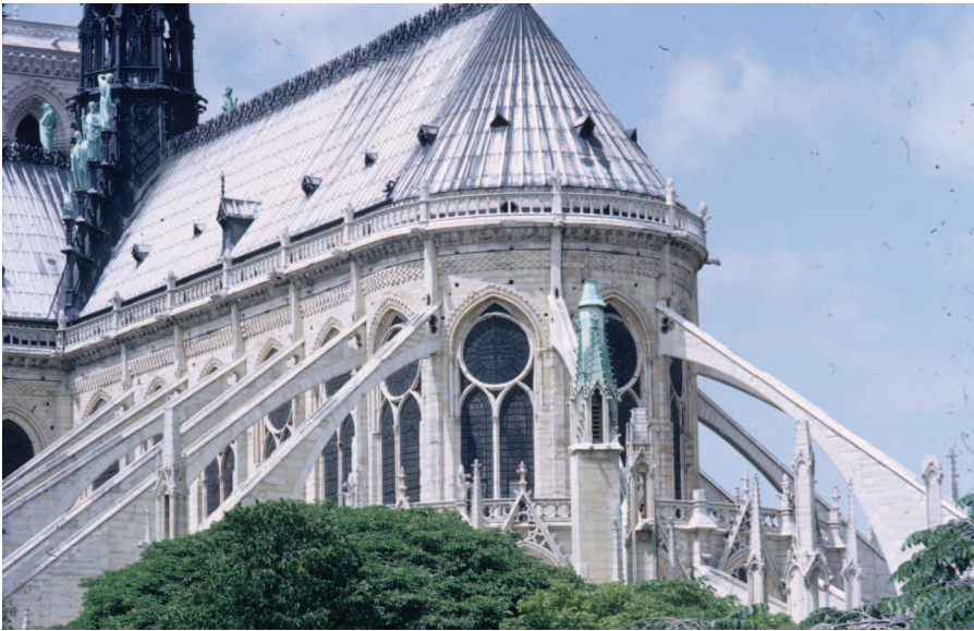
Figure 1 "Looking at a gothic church, you never get tired, you will never be finished with it.": East end flying buttresses of Notre Dame Cathedral, Paris, 1163 AD. (PD 693).
