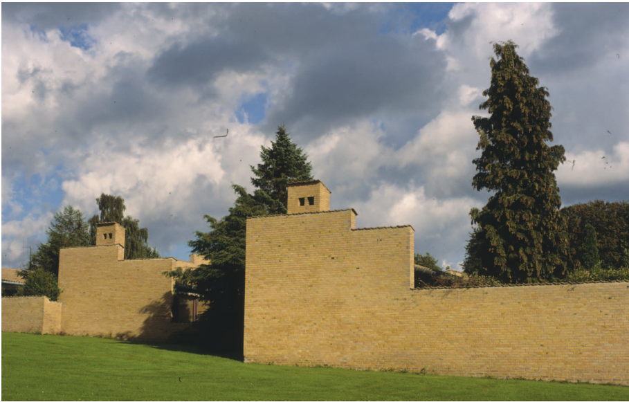
Figure 7 Utzon's interest in the primitive found an outlet in his adoption of the ancient Chinese courtyard house type as the basis for a series of housing experiments, namely the Kingobusene Housing Estate outside Helsingør, 1957-1960, and later, in the luxury Fredensbørg housing, 1962-1963, illustrated. The repetition of variations of the same plan type anticipated Utzon's later theory of additive architecture. (PD 15 549).
